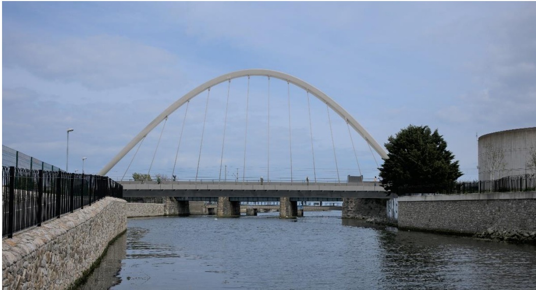
Figure 3. Proposed Bow String Arch Bridge
